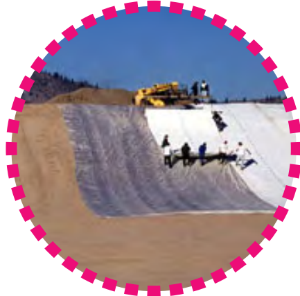
4. BENTONITE CLAY LINER
