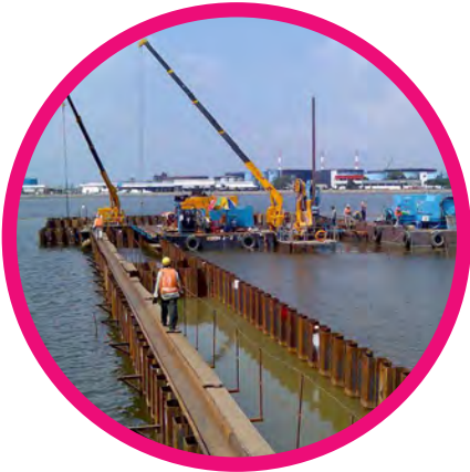
1. CRIBBING + SEALED SHEETPILES
