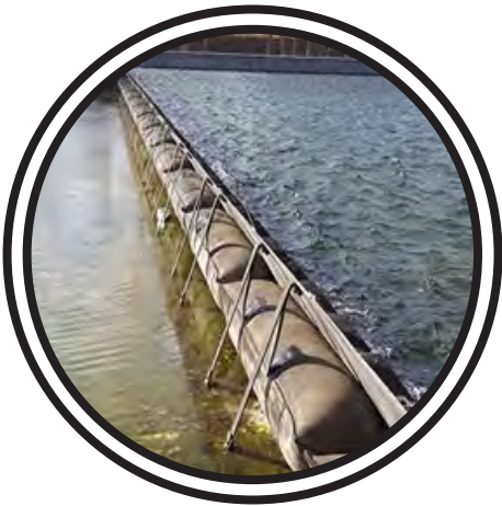
3. INFLATABLE BARRIER
